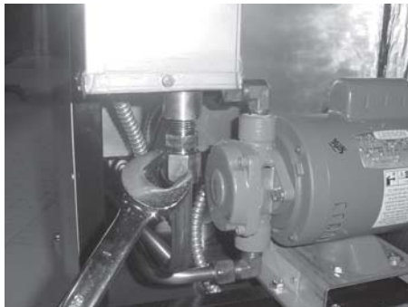
Condensation Box Fitting Step 1
